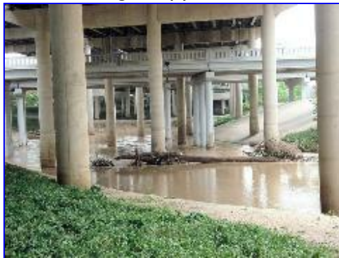
Logjam at I-45 - High water on April 30, 2009 created a logjam near I-45 and Rusk Avenue that completely obstructs the channel.
